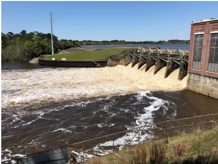
View of the Lake Talquin Dam at Jackson Bluff.
